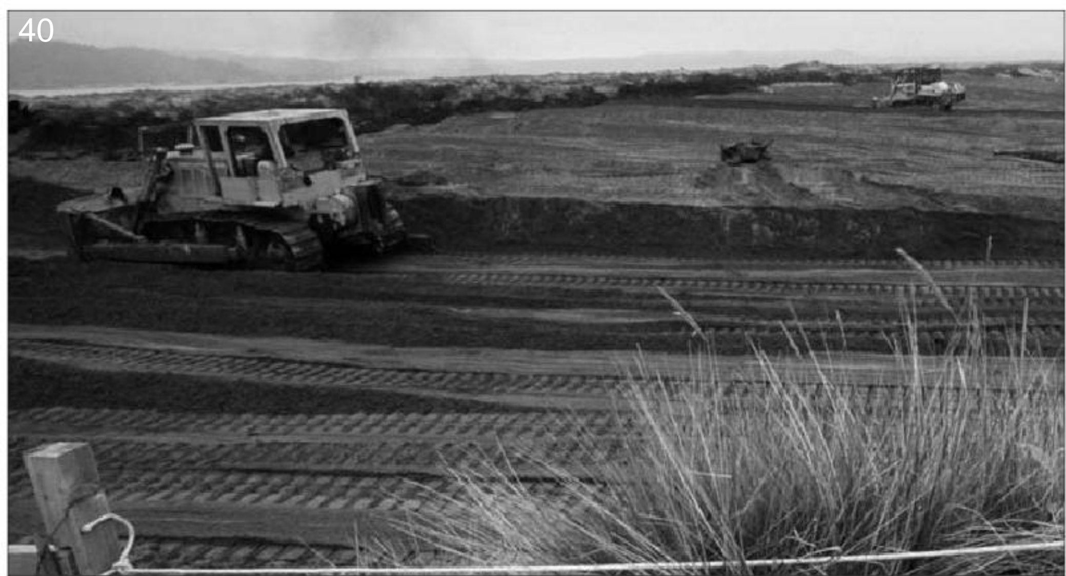
Fig. 8. Bulldozers removing Ammophila arenaria for a western snowy plover habitat restoration project at the South Spit, managed by the Bureau of Land Management (beachgrass was first burned to reduce biomass).
